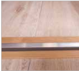
oak threshold for wooden door frame
