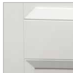
chamfered connection of rails and stiles
